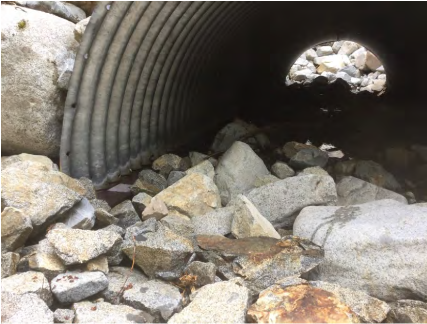
Consistent bearing on both footings, right bank shown
